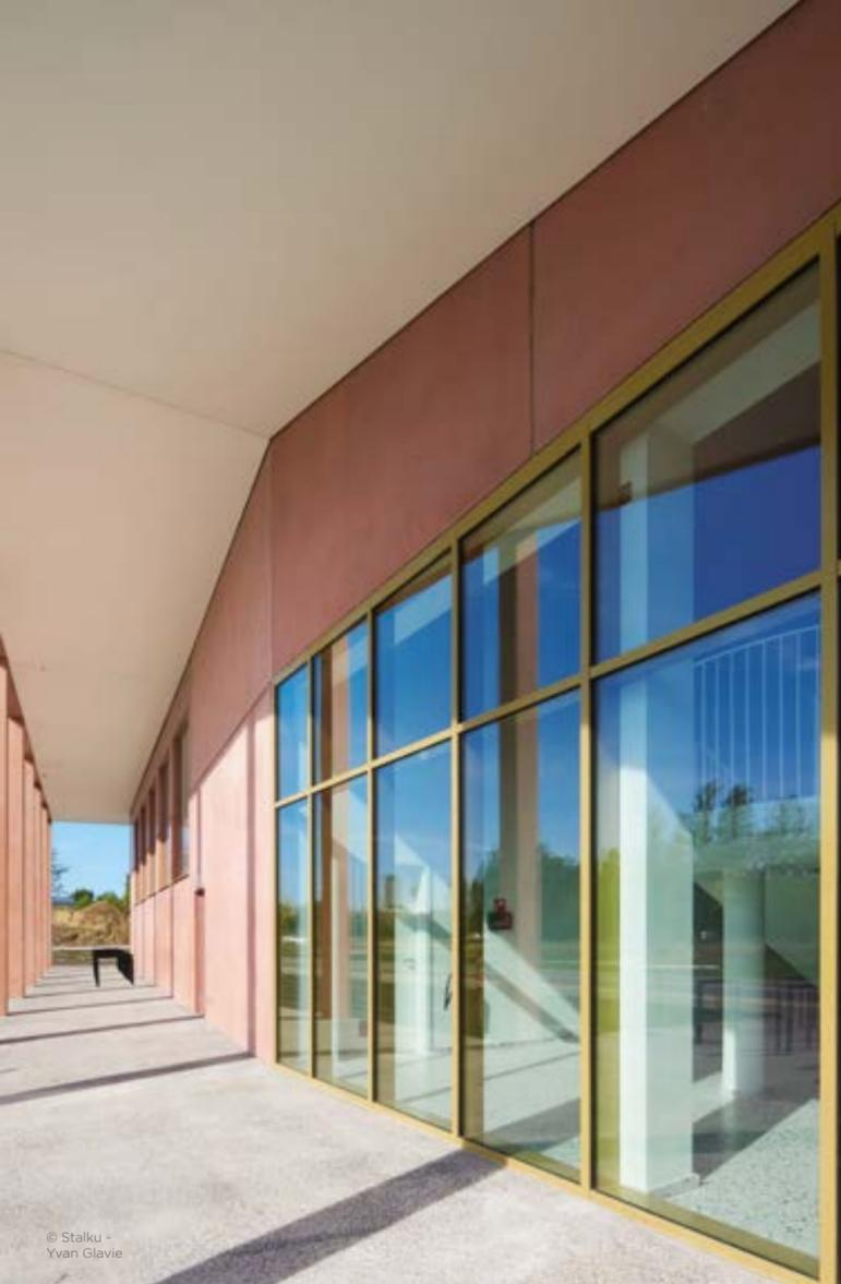
The **MC WALL** executed as a traditional curtain wall has a wide choice of clamp and cover profiles as an aesthetic finish. Style profiles are available up to a depth of 326 mm. Because we extrude at lengths of 7 metres as standard, a free span can be created in almost all situations without using a slide-in profile. A wide choice of profiles makes it possible to bring the posts and rails into one plane on the inside.
